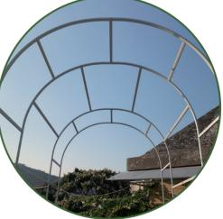
Install twenty-two D-rod support rods on both sides, one rod at every other hole until the top.
