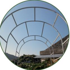
Install twenty-two E-rod support rods on both sides, one rod at every other hole until the top.
